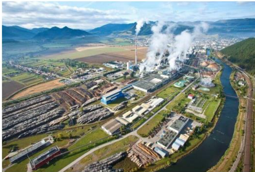
Mondi SCP Plant overview (Source: https://www.profisteelholding.sk/en/reference/mondi-scp-2/ )
