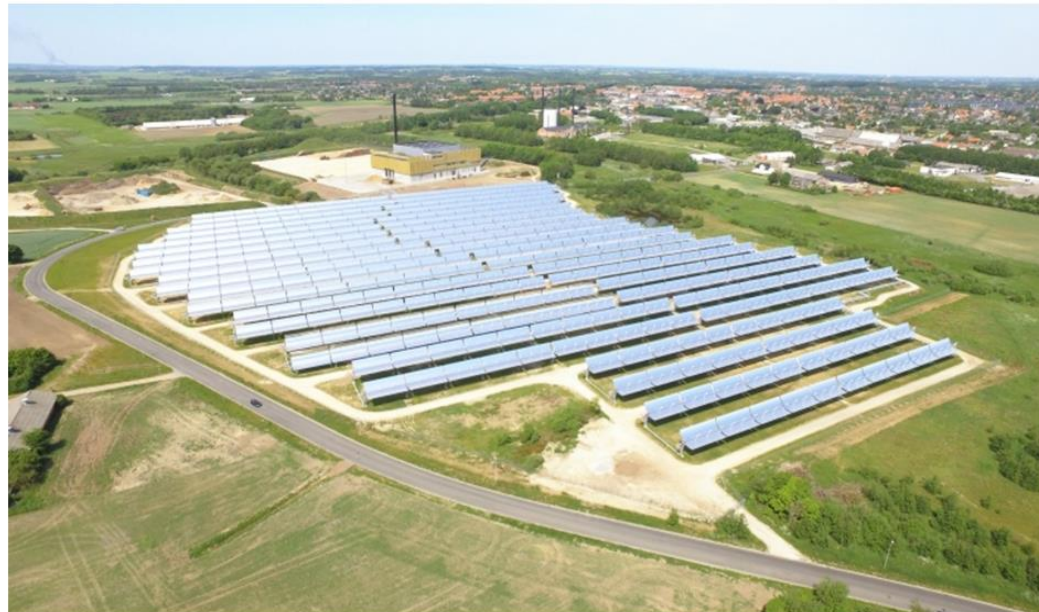
Brønderslev Full plant overview (solar field)
